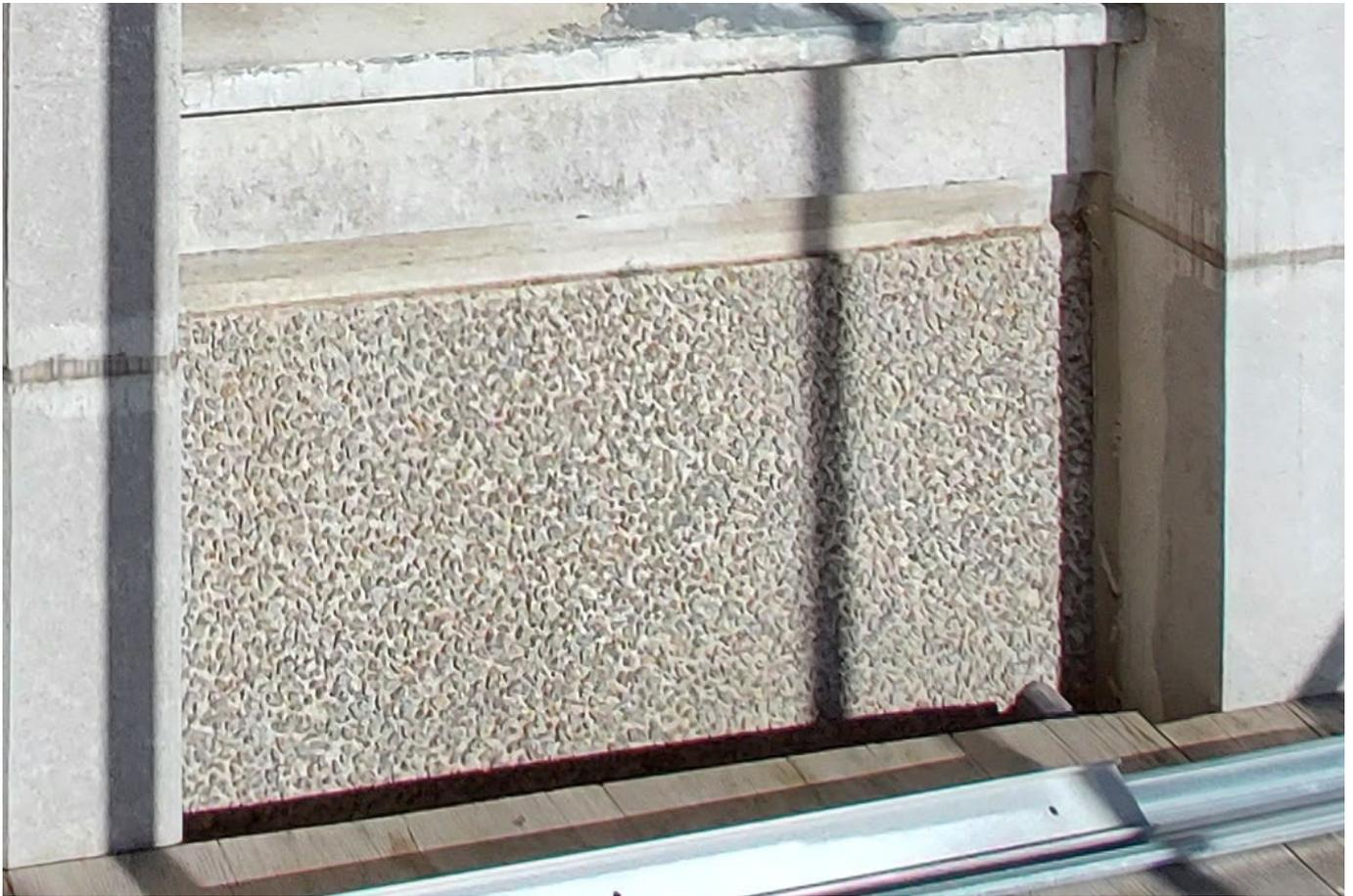
I used a SDS-X-6.0\*210-P drill bit (rebar drill) with hammer action as the pebble render makes it more difficult to drill with a SDS-P-6.0\*210-P standard drill bit.
