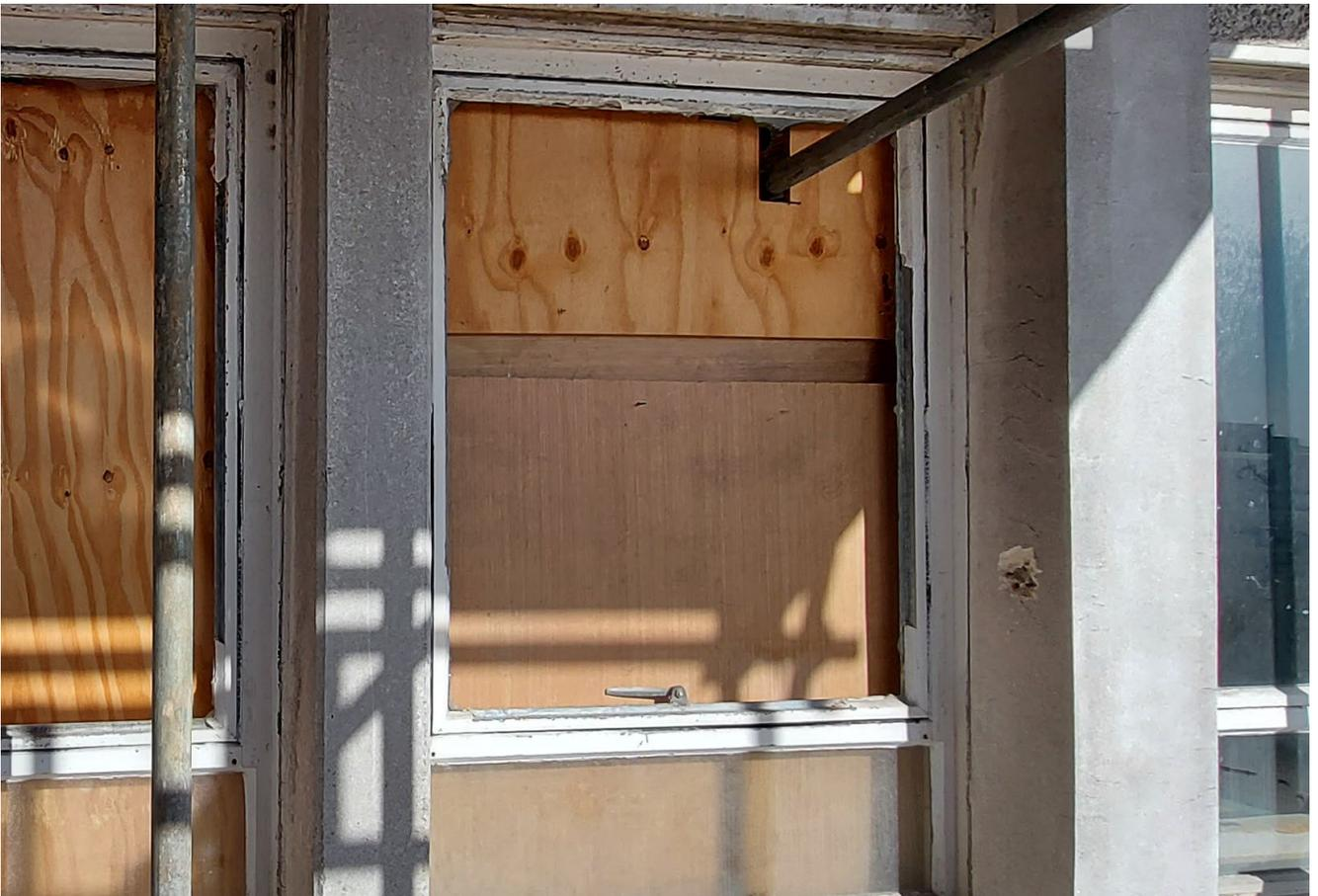
I was able to drill the concrete with a standard SDS drill bit – SDS-P-6.0\*210-P – hammer action was required.
